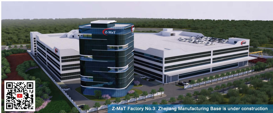
Z-MaT Factory No.3: Zhejiang Manufacturing Base is under construction
