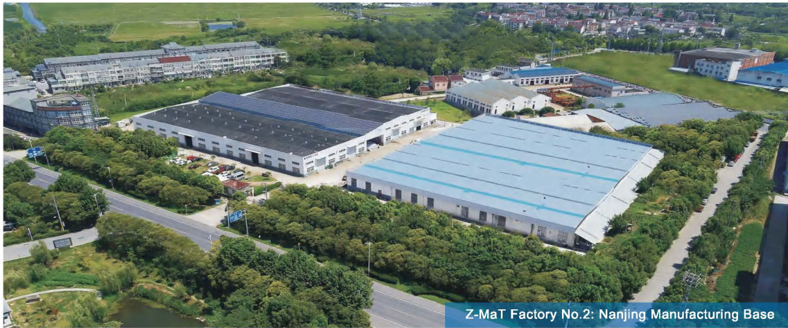
Z-MaT Factory No.2: Nanjing Manufacturing Base
